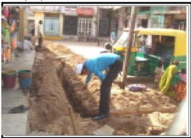
Laying drainage pipe at Kapadvanj Nagarpalika
